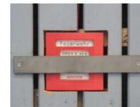
Brandmelder in Halle
